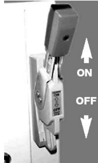
Figure 2.18 - Main Circuit Breaker Switch
